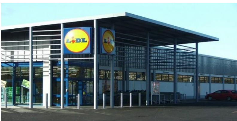
Logistic Center in the Industrial Area of Thessaloniki.
