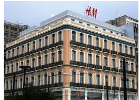
H&M building in Piraeus
